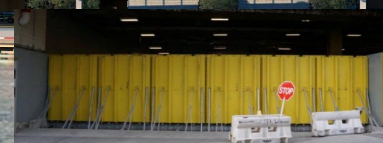
LOADING DOCK DEPLOYABLE FLOOD GATE
